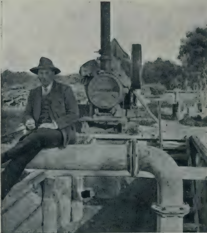
Pumping Plant in use on Moorara Station, on the Darling.
